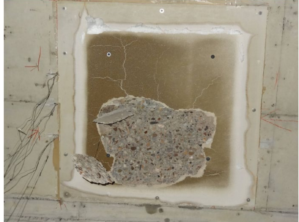
After fire test
