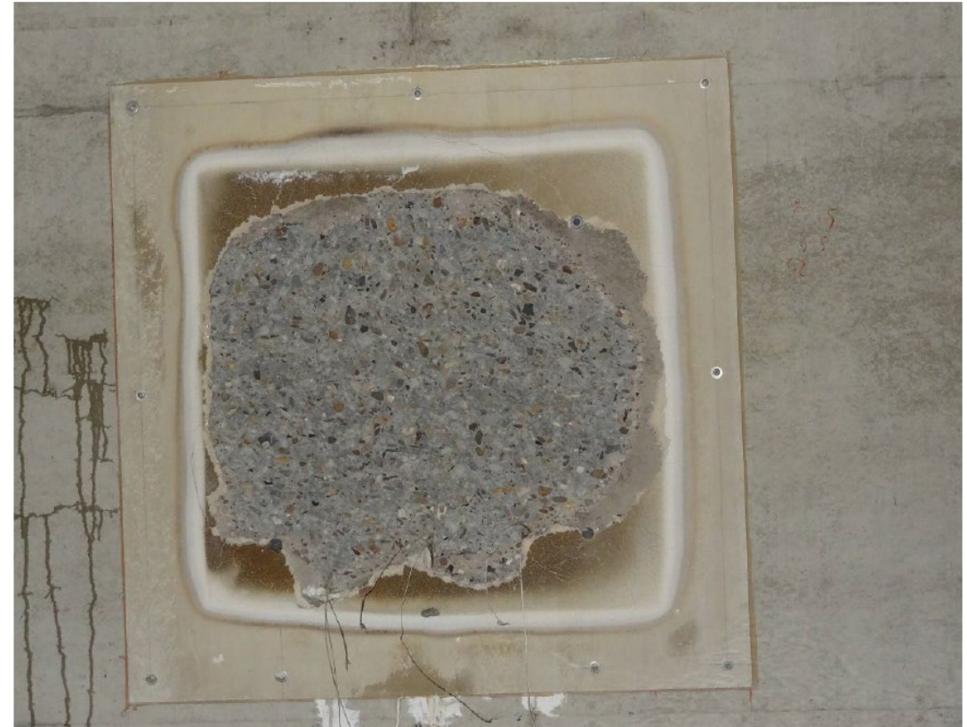
After fire test
