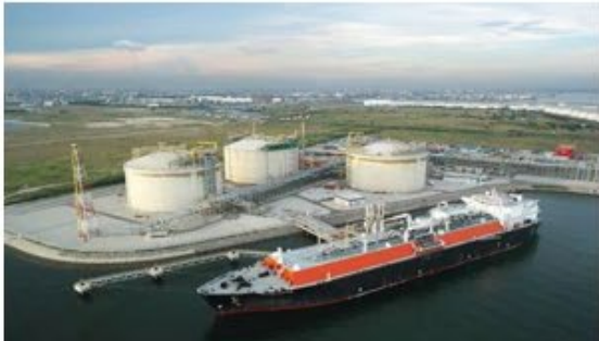
LNG/LPG Terminal (Onshore)
