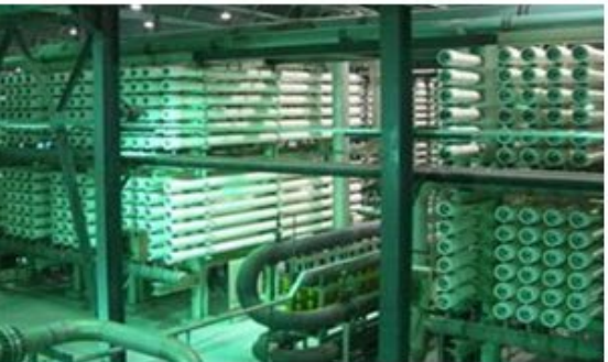
Water Treatment Plant
